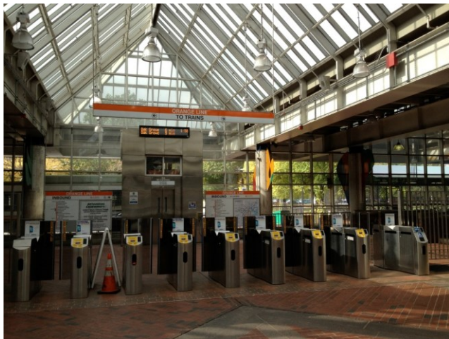
Photo 5-5b. Subway turnstile (entrance/exit)
